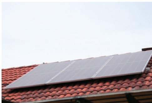
SOLAR PANEL INSTALLATION AND MONITORING
